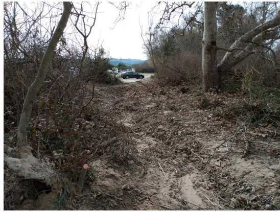
Photo: Mud and debris flow with vegetation clearing between bridge and parking area. Photo by Michele Jimenez-Holtz.
