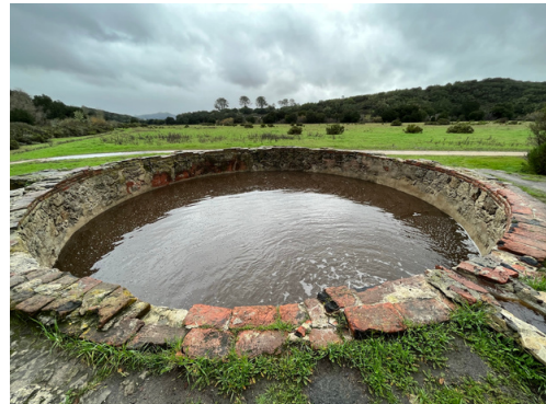
Photo: Full cistern during January storms.
